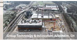
Group Technology & Innovation, Aulesheim, CH
